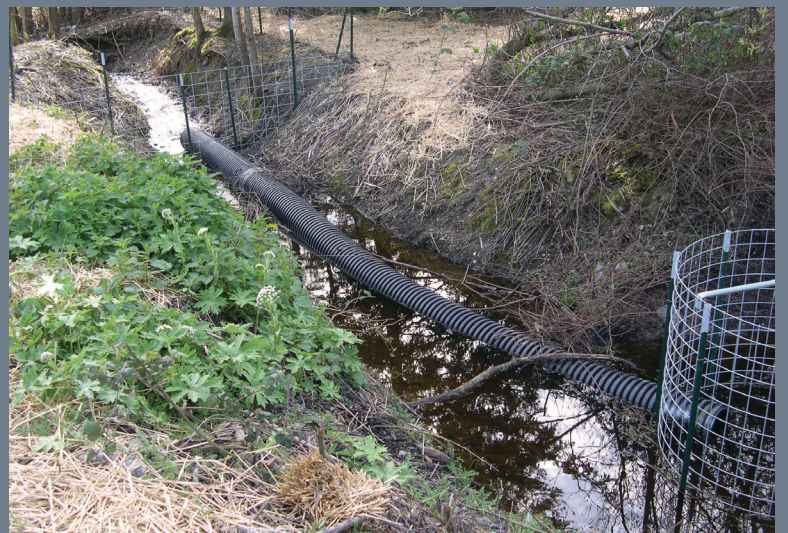
View the beaver pond, leveler and deceiver at the NW corner of East Camano Drive and Can Ku Rd. There are signs and a viewing platform.
