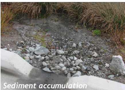
Excessive ponding - clogged overflow
